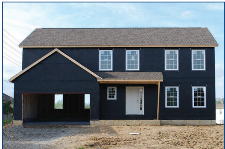
AFTER Sheathing system is completely protected against liquid moisture, moisture vapor and uncontrolled air leaks
