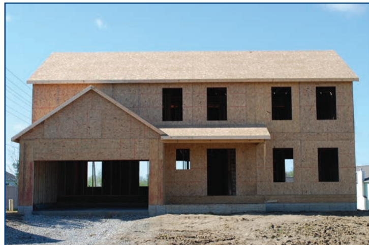
BEFORE Sheathing system is exposed to moisture, air leakage and the elements allowing water to penetrate and air to leak through the seams.
